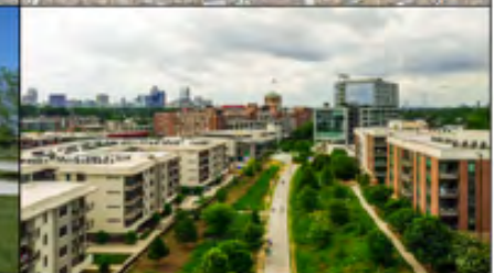
Atlanta, GA Repurposed Rail Corridor 3 miles long, average 120-foot width Part of a citywide multi-modal ring trail
