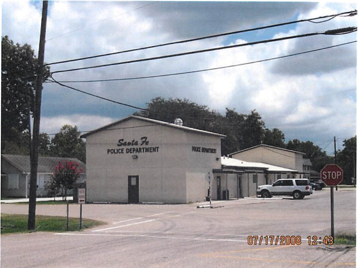
Existing Santa Fe Police and Courts Building
