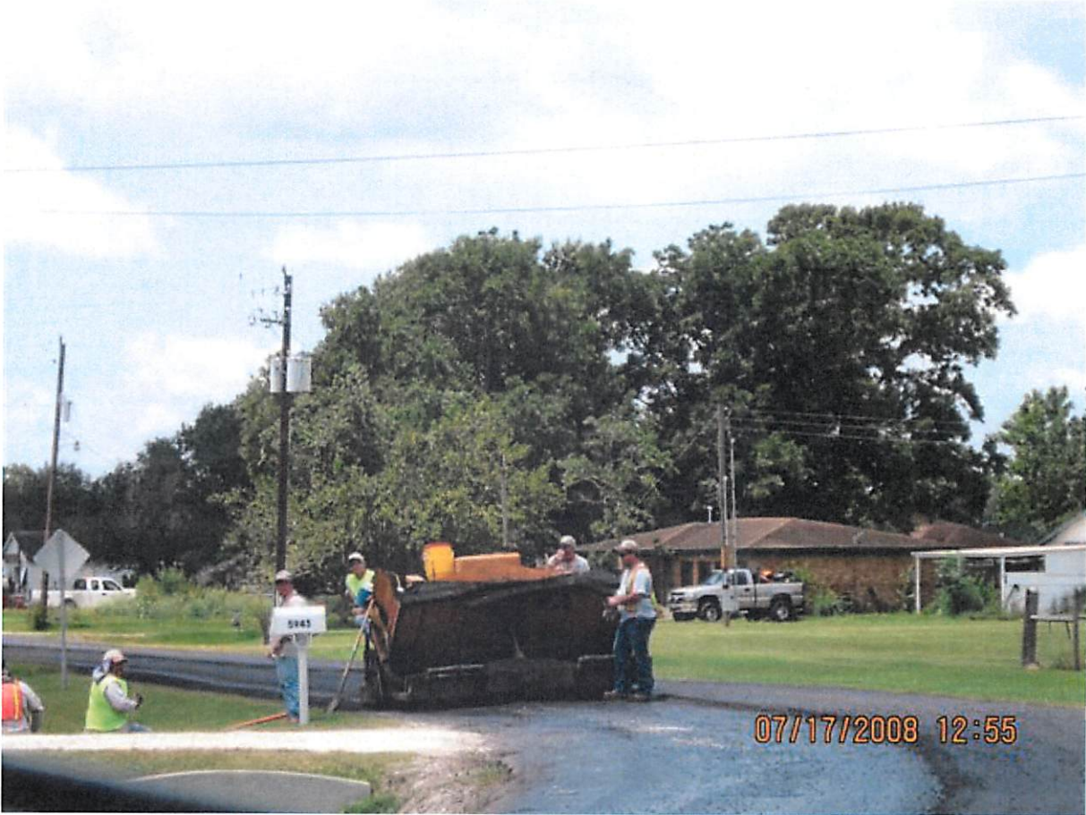
Asphalt Paving in the City of Santa Fe
