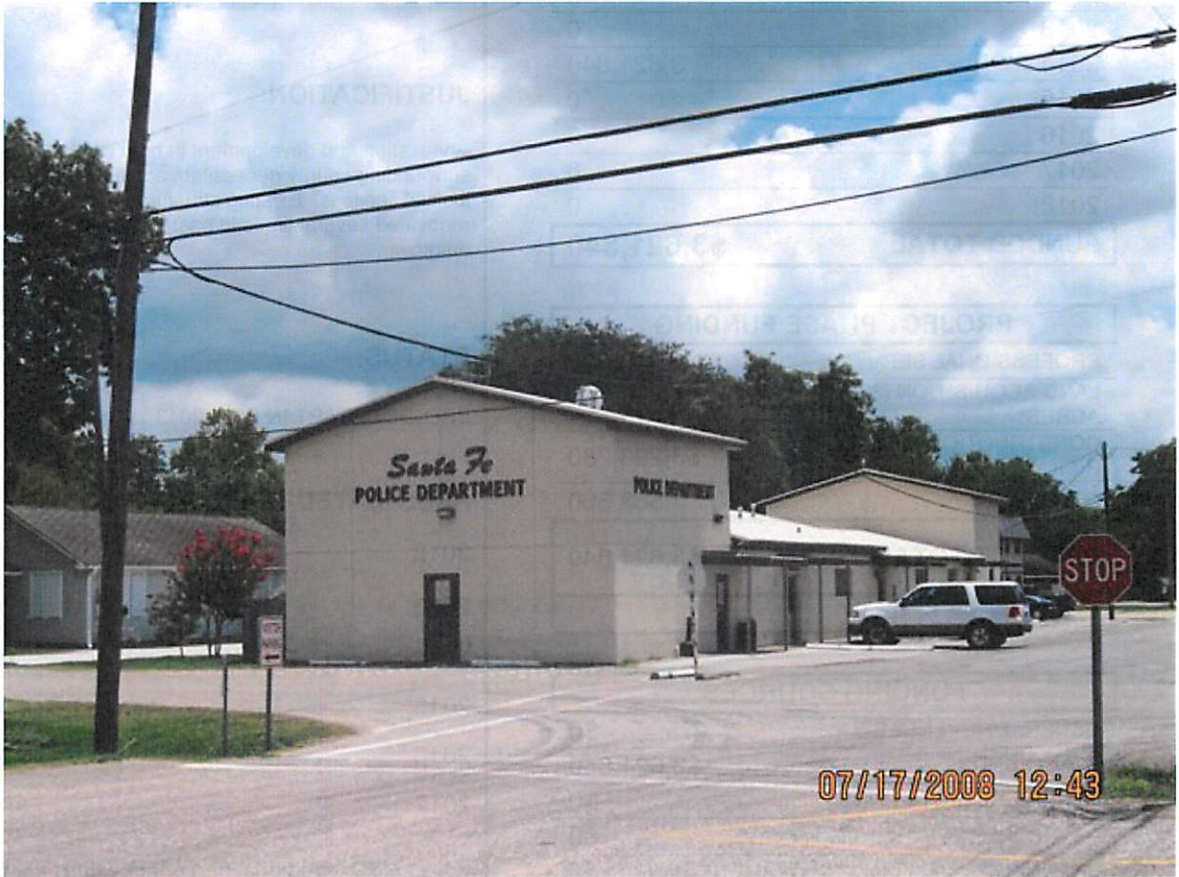
Existing Santa Fe Police and Courts Building
