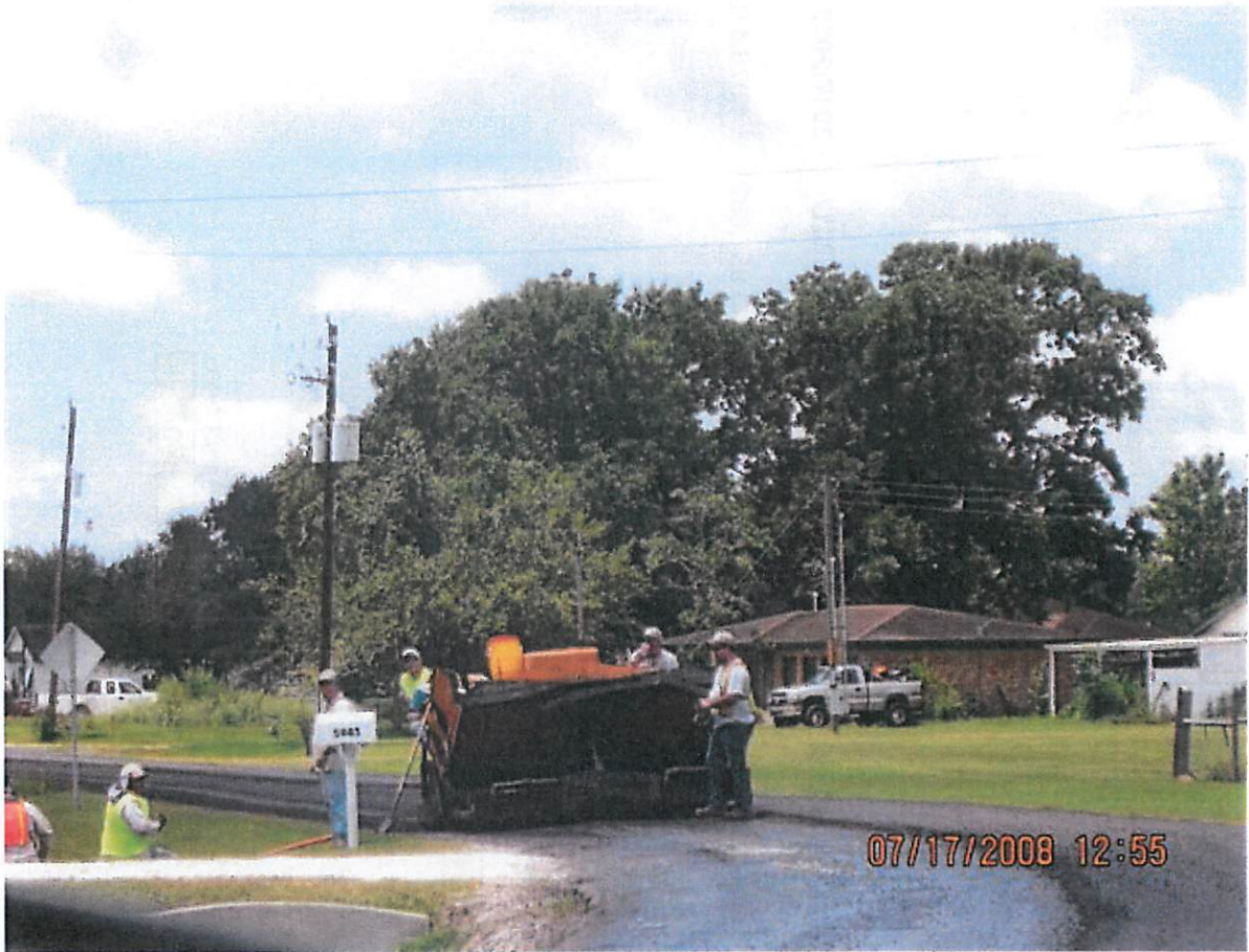
Asphalt Paving in the City of Santa Fe
