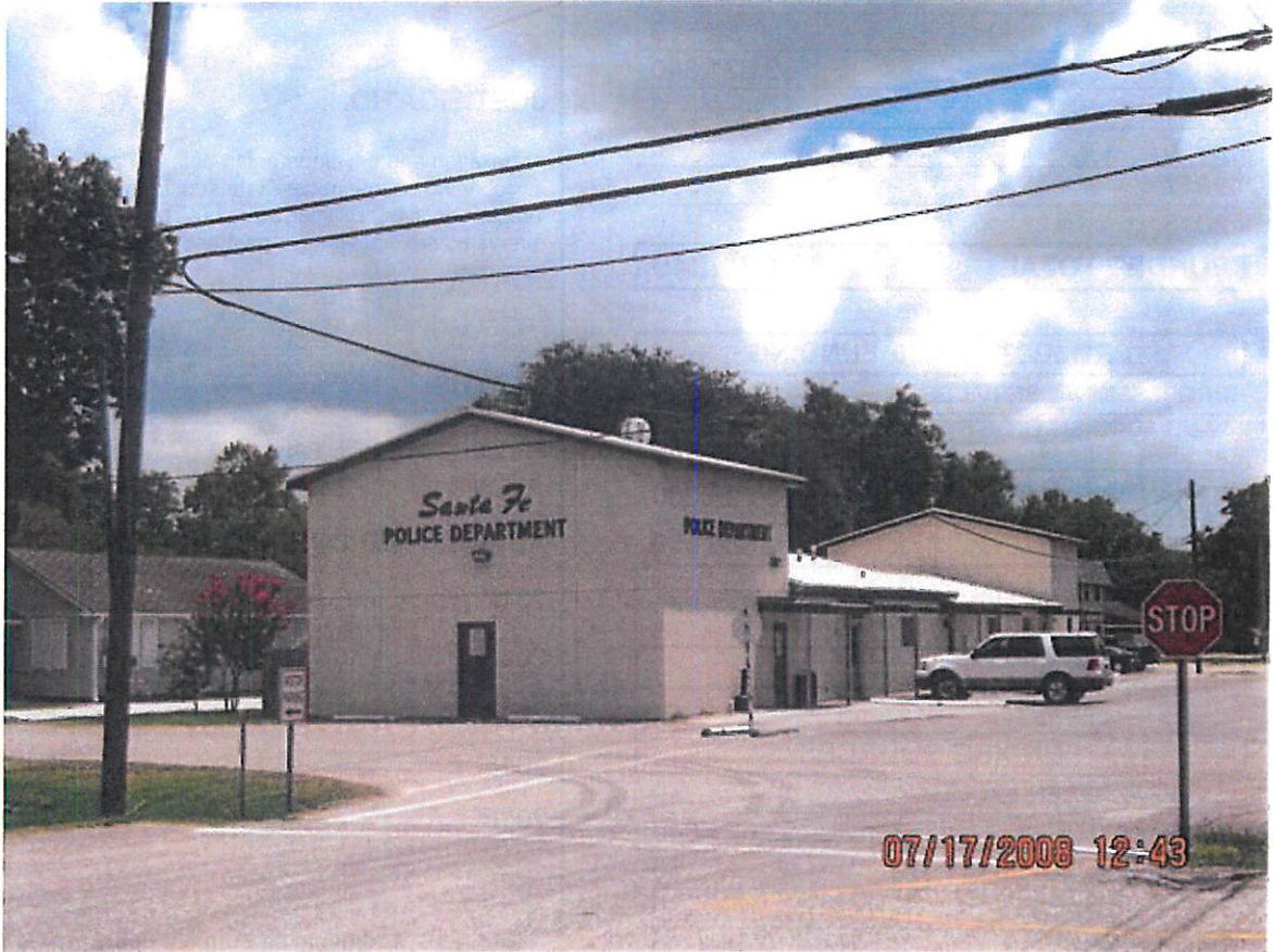
Existing Santa Fe Police and Courts Building
