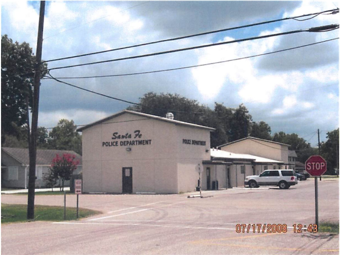
Existing Santa Fe Police and Courts Building
